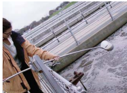
A wastewater treatment plant.
